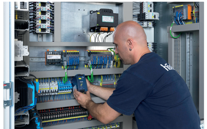
Control panel construction
